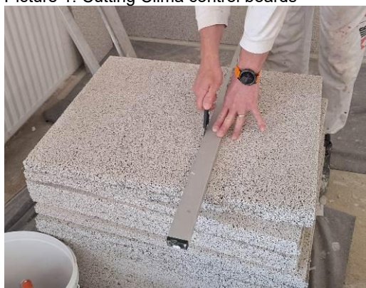
Picture 1: Cutting Clima control boards
